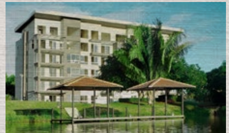
LAKUS 1 tower with 20 apartments with view
