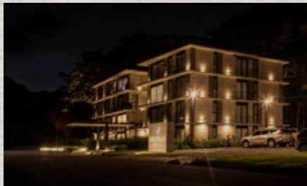
NAUTILUS 2 towers with 16 apartments each
